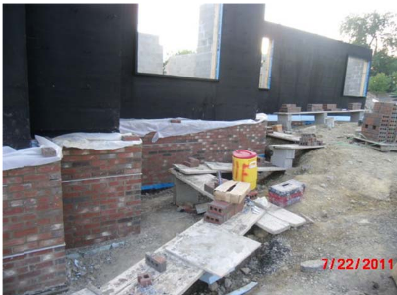
(Figure 1: Façade Irregularity)
